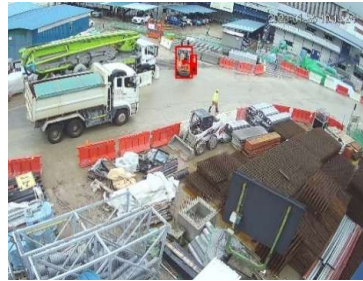
3. Worker near vehicles/ heavy machinery
